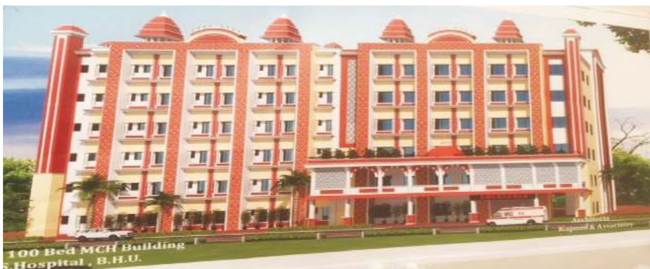
100 Bed MCH Building, S.S. Hospital
